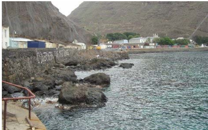
Fig 9 - Area for development at Jamestown Port
