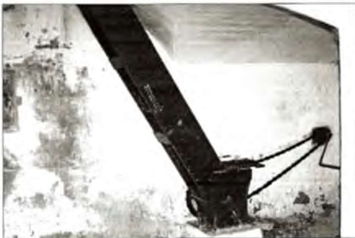
Shell hoist for the 6-inch guns.
